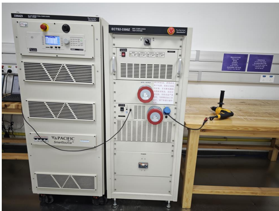
Photograph 6: Set-up for Harmonics, Voltage Fluctuation and flicker
